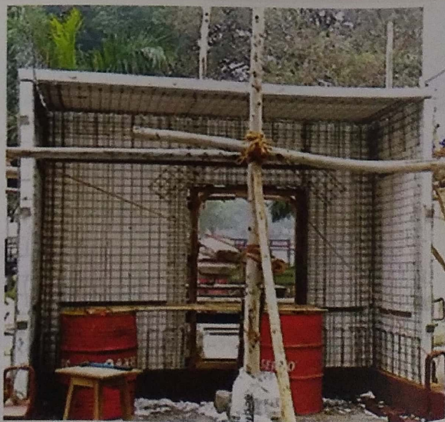
Building skeleton made of factory-made EPS core panels
